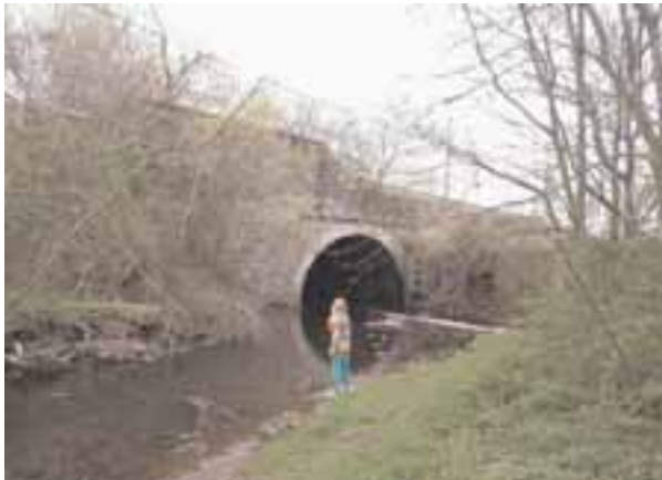
Sawmill Run arch culvert adjacent to MLK Park
